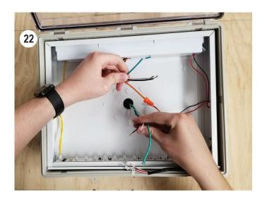
19. With the proper connections made, conceal the wires inside the J-box (all power supply wire connections need to be made inside the J-box). Snap on battery compartment until the tabs are locked and secured to prevent interference with the EXIT sign illumination. (Fig. 23 and 24)
