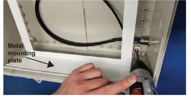
3. Using the supplied enclosure mounting template on Page 11, choose the necessary holes for the J-box. (Fig. 4)
