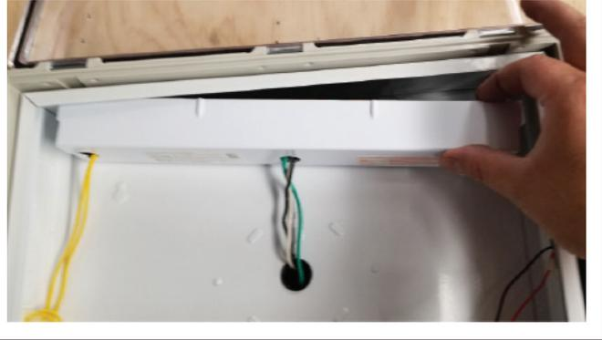
21. Locate the battery wire coming from the battery compartment and plug the connector into the PCBA connector at the location shown. The PCBA connector for the battery is located behind the connector for the test switch, labeled "TEST" (Fig. 23 and 23a)
